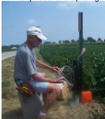
Bud Link splicing cable along St. Anthony Rd.
